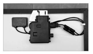
**TIPS & TRICKS:** Twisting the PV module wires and/or tying a loose knot can also help manage these wires.
