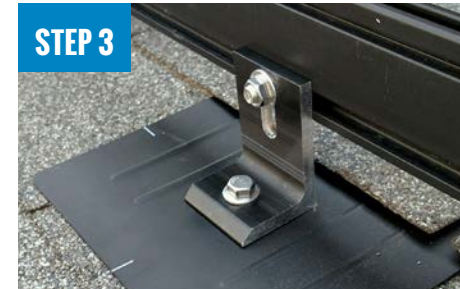
ATTACH L-FOOT TO RAIL
