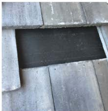
1 Remove tiles around installation area
