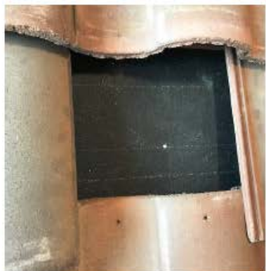
2 Locate, identify, and mark the rafters.
