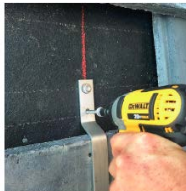
5 Reposition the hook and secure using included lag screws
