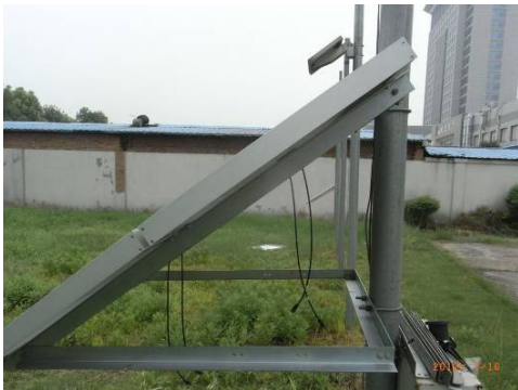
安装好的组件和支架 Photo of Assembled Mount.
