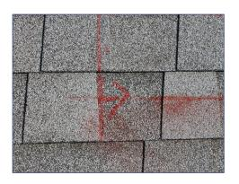
2 Using locations drawn on roof during system layout, drill a 3/16" pilot hole into roof framing member.
