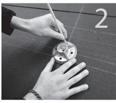
Align QBase vertical holes over center rafter mark and horizontal holes over snapped line. Mark holes for drilling.
