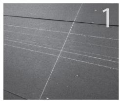
Layout your array out over the roofing paper using a chalk line to mark rafter centers and the rail location center.
