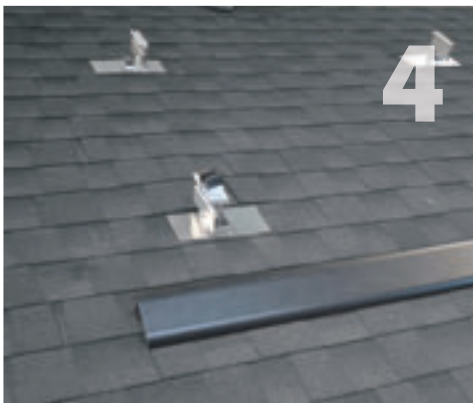
Match the skirt cantilever to the module cantilever based on your array design.
