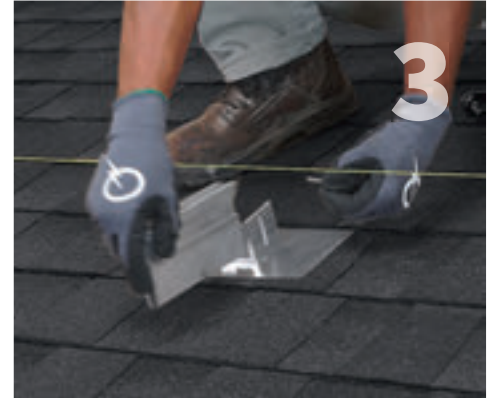
3 To adjust in 1/4" increments move the top slider up or down one notch. To adjust in 1/8" increments rotate the top slider 180 degrees. Repeat for the other mounts until top slider elevations are uniform across the row.
