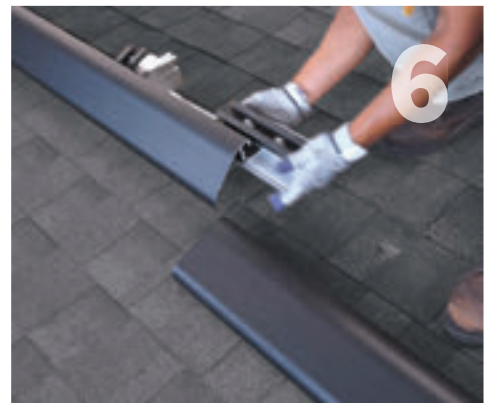
Slide 8" bridge clamps onto the skirt segments at the module intersections. Slide the clamp about halfway onto one side of the skirt, and then slide the next segment of the skirt onto the other side of the clamp, finishing by sliding the skirts flush together.
