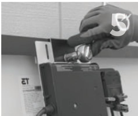
5 Tighten the cap screw with a half-inch socket and torque wrench. Torque to 15 foot-pounds.
