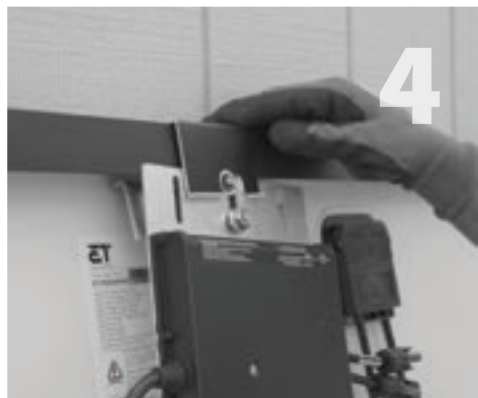
4 Slide the entire unit up under the bracket clamp, and then slightly to the left so that the cap screw holds everything together.
