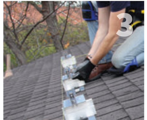
Align first row of clamps using a string line. Tighten all aligned first row clamps using the 1/2" open end wrench.
