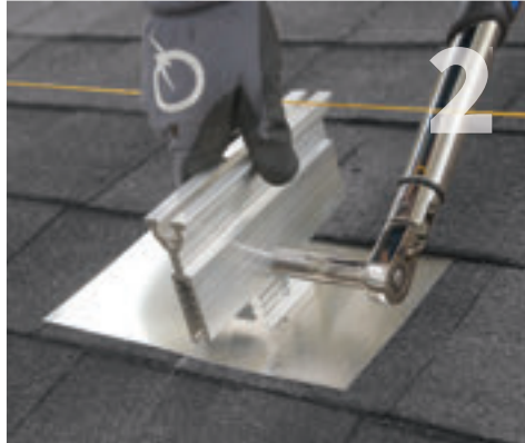
2 The string acts as a guide for aligning the top slider positions of all the mounts in the row. To adjust top slider height, remove machine bolt, separate top slider from QBlock slider and reinsert at proper location. Use torque wrench 1/2" socket to torque all top slider bolts to 6 ft-lbs.
