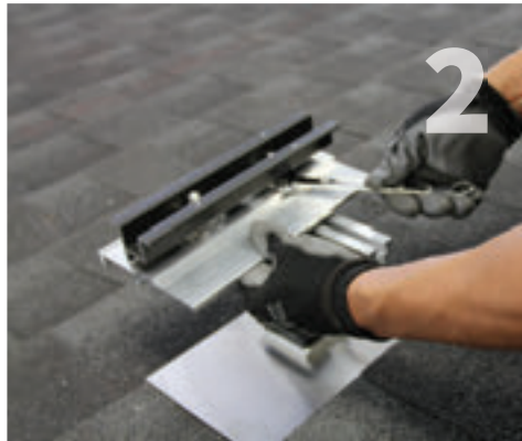
Use 1/2" open end wrench on mid-clamp assembly nut to tighten clamps to first and last (far left and right) top sliders.
