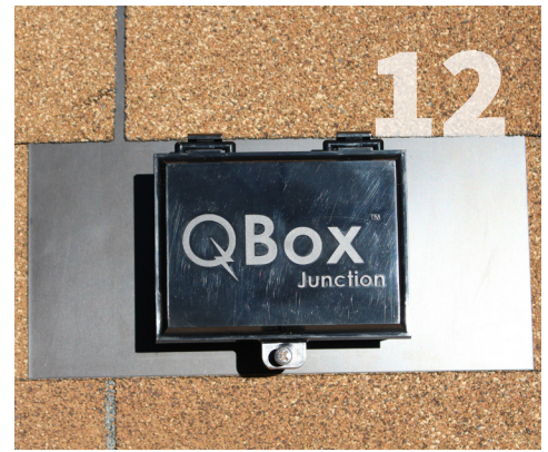
Close Lid: Close and thread the bolt into the nut by hand. Then using a #3 Philips drive, turn bolt until the top and bottom tabs securing the bolt are flush.
