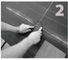
Lay out your array over the felt paper using a chalk Using the QBase as a guide, mark pilot hole location for drilling. If roof is already felted, cut a section in the topmost layer for the QBase, so that the shakes underneath can still slip under the felt.
