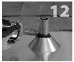
Apply a bead of sealant around the area where the cone flashing meets the post.
