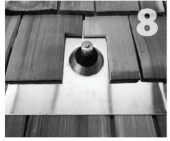
The mount installation is now complete. Continue roofing around the mount assembly, cutting shakes to accommodate the flashing cone.
