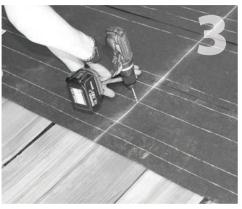
Drill 2 each 7/32" pilot holes into rafter. Do not use QBase as a drill guide. Hold drill square to rafter. Fill pilot holes with sealant compatible with roofing material.
