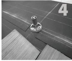
Prior to mounting to the roof, seat the grade-8 bolt (item 1) through bottom of QBase, and screw post (item 6) into base. Place QBase with post over drilled holes and secure lags (item 3) in place. Tighten to a snug fit.
