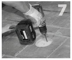
Using QBase (item 2) as a guide, align two clearance holes vertically with the center of the rafter. Mark the center of these 2 holes. Drill 7/32" pilot hole at each of the 2 marks. Hold drill square to rafter. Do not use QBase as a drill quide.
