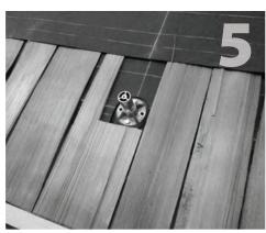
Roofing now continues. Cut shakes as needed to accommodate the QBase.
