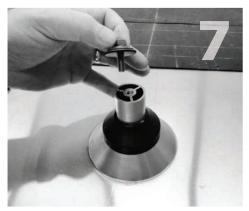
Apply a bead of sealant around the area where the cone flashing meets the post. Install the EPDM rubber counter flashing (item 5) over the post, and attach all the remaining hardware (items 7-10) on top of the post for safekeeping until the racking is ready to install.
