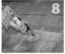
Fill pilot holes with sealant compatible with roofing material such as Chemlink M-1, Geogreen 4500, or Solar Seal 900.
