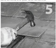
To remove the slate below the score, slightly lift Using a 4" diameter diamond hole saw and the the lower portion of slate with a slate ripper, then pilot hole drilled in step 3, drill through the existing gently but firmly tap the top piece with a hammer. slate. The lower piece should break off cleanly.
