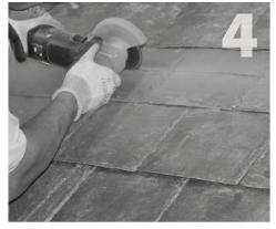
Using a cutoff wheel in a grinder, score the slate above the mounting area at 4 inches above the center of the QBase location. In step 5, you will remove the slate below the score line, which will allow you to slide the flashing up under the remaining slate in step 10.
