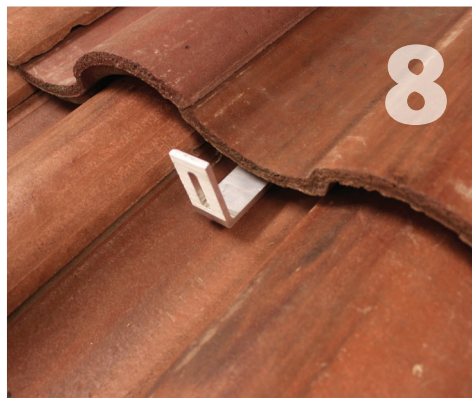
Bolt the side-mounted rail of your choice to the hook, using the rail manufacturer's hardware.
