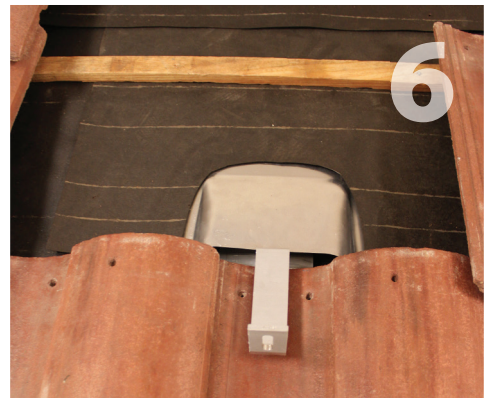
Quick Mount PV recommends installation per the Tile Roofing Institute guidelines with a base flashing. Alternative flashing methods may be approved by the AHJ at their discretion.
