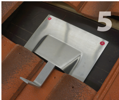
Carefully clean the underlayment then apply bead of sealant compatible with roofing materials in the shape of an upside down U on the backside of the sub-flashing, and install flashing over mount. Fasten sub-flashing to deck with one roofing nail in each top corner. Do not nail bottom corners.
