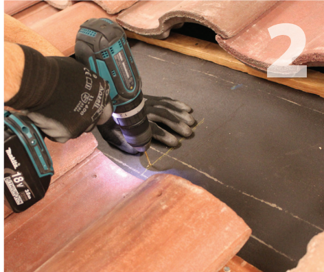
Rest the base plate over center of rafter and mark center of holes. Drill two 7/32" pilot holes and fill with sealant compatible with roofing materials.
