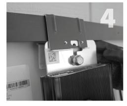
Slide this assembly onto the module frame with the bracket behind the module frame, the module level electronic mounting bracket in front of the module frame, and the bracket clamp in front of the module level electronic mounting bracket. Slide the assembly up and to the left to engage cap screw into bracket clamp slot.
