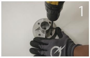
Locate the desired mount placement per the plan set. The mount can be attached to structural members or direct to the roof deck based on site-specific criteria. Using the base as a template, mark the penetration points with either a pen or light drilling. When attaching to a structural member, use two opposing holes on the base plate, parallel to the structural member.
