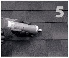
Clean off any sawdust, and fill hole with sealant compatible with roofing materials.
