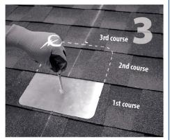
Insert flashing between 1st and 2nd course. Slide up so top edge of flashing is at least ¾" higher than the butt-edge of the 3rd course and lower flashing edge is above the butt-edge of 1st course. Mark center for drilling.
