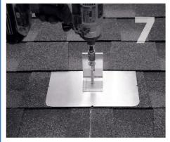
Prepare lag bolt or structural screw with sealing washer. Using a ½-inch socket on an impact gun, drive prepared lag bolt through L-foot until L-foot can no longer easily rotate. **DO NOT over-torque.** NOTE: Structural screw can be driven with T-30 hex head bit.
