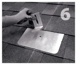
Place L-foot onto elevated flute and rotate L-foot to desired orientation.
