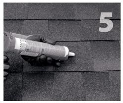
Clean off any sawdust, and fill hole with sealant compatible with roofing materials.
