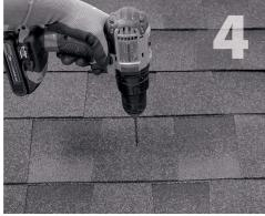
If attaching with lag bolt use a 1/4" bit (Lag). Use a  $\frac{1}{2}$ " bit (ST) for attaching with the structural screw. Drill pilot hole into roof and raft er, taking care to drill square to the roof. Do not use mount as a drill guide. Drill a 2" deep hole into
