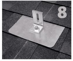
You are now ready for the rack of your choice. Follow all the directions of the rack manufacturer as well as the module manufacturer. NOTE: Make sure top of L-Foot makes solid contact with racking. All roofing manufacturers' written instructions must also be followed by anyone modifying a roof system. Consult the roof manufacturer's specs and instructions prior to working on the roof.
