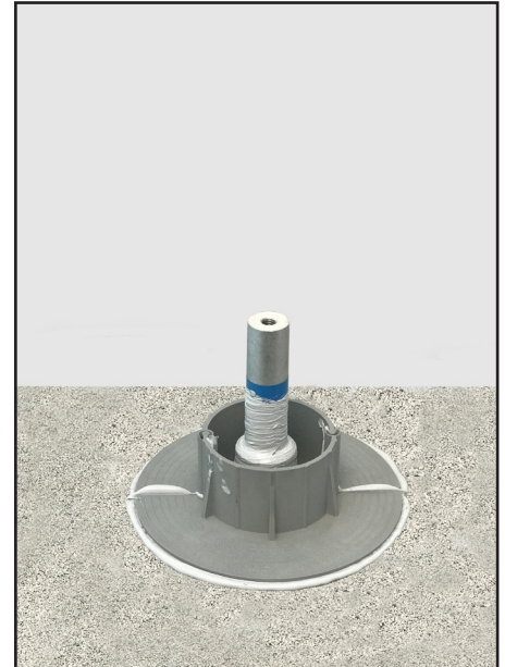
STEP 4: Adhere E-Curb to roof surface.
