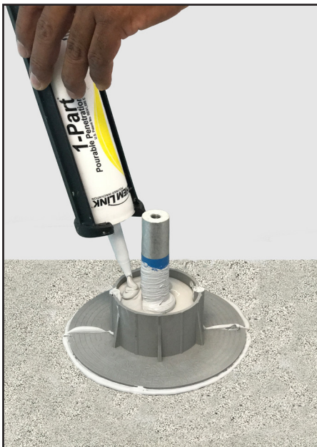
STEP 5: Fill E-Curb with 1-Part filler and remove tape.
