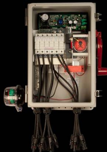
Pre-wired Disconnecting PV Combiner - MNPV6HV-MC4
