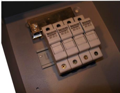
4 Touch safe fuseholders installed in an MNPV6
