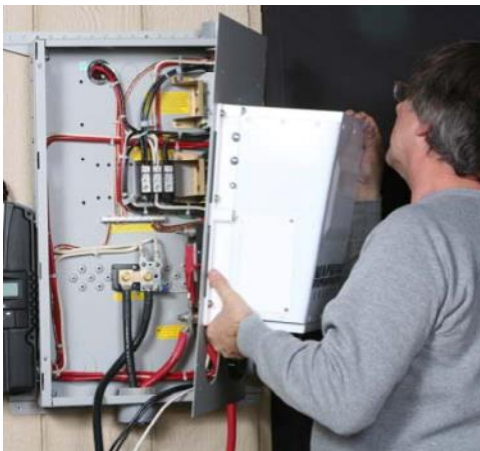
Figure 9, Lifting the door into the E-Panel hinge openings
