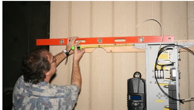
Measuring and marking before mounting the MNDC-X2 to the wall.
