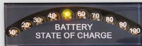
Batteries have a 50% charge
