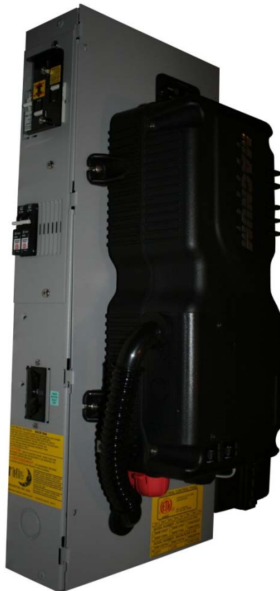
E-PANEL FOR MAGNUM MM SERIES AS INSTALLED
