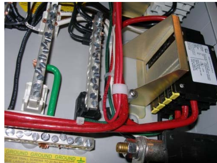
Ground to Neutral connection
