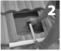
Use a straight edge and measure up 6 %" from bottom of tiles to center of the mount over the center of rafter.
