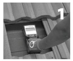
Remove tile. Locate and mark center of rafter.
