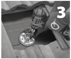
Align QBase over rafter center and drill two ½2" pilot holes. Fill pilot holes with sealant compatible with roofing material. Place grade-8 cap screw under QBase in hex slot, threads pointing up. Lag QBase into rafter through pilot holes.
