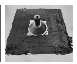
**NOTE:** The TRI/FRSA Florida guidelines indicate the sub-flashing being flashed using the three-course method on ALL FOUR SIDES. Alternative flashing methods may be approved by the AHJ at their discretion.
