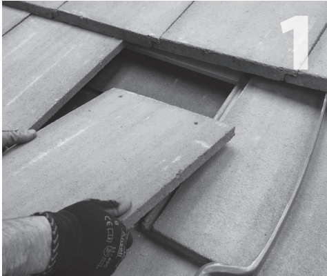
Remove tile at selected location of mount.
