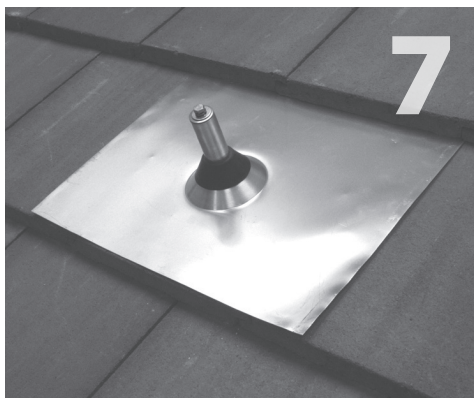
Apply sealant where post and flashing meet, and install counter flashing collar. (Be sure to seal off the post from weather exposure with the sealing washer, in the interim before racks are installed.)
