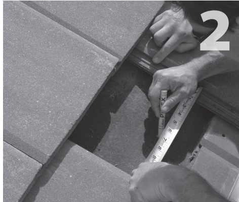
Locate and mark center of rafter.
