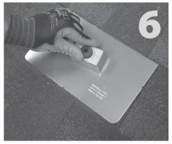
Slide the flashing into position. Insert the rubber plug into the QBlock cavity.
