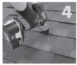
Using drill with 7/32" bit, drill pilot hole into roof and rafter, taking care to drill square to the roof. Do not use mount as a drill guide. Drill should be 'long style bit', aka 'aircraft extension bit' to drill a 1¾" deep hole into rafter.
