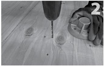
Drill both pilot holes with a 7/32-inch bit. Make sure to hold the drill square to the rafter. The lag bolts must be anchored into a structural member, so it is very important to hit the center of the rafter with your pilot holes. Fill the pilot holes with a sealant compatible with roofing materials.
