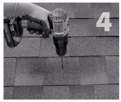
If attaching with lag bolt use a 7/32" bit (Lag). Use a 1/8" bit (ST) for attaching with the structural screw. Drill pilot hole into roof and rafter, taking care to drill square to the roof. Do not use mount as a drill guide. Drill a 2" deep hole into rafter.
