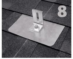
You are now ready for the rack of your choice. Follow all the directions of the rack manufacturer as well as the module manufacturer. NOTE: Make sure top of L-Foot makes solid contact with racking.
