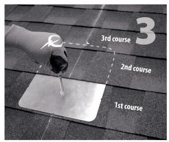
Insert flashing between 1st and 2nd course. Slide up so top edge of flashing is at least ¾" higher than the butt-edge of the 3rd course and lower flashing edge is above the butt-edge of 1st course. Mark center for drilling.
