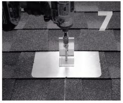
Prepare lag bolt or structural screw with sealing washer. Using a ½-inch socket on an impact gun, drive prepared lag bolt through L-foot until L-foot can no longer easily rotate. **DO NOT over-torque.** NOTE: Structural screw can be driven with T-30 hex head bit.
