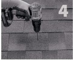
If attaching with lag bolt use a  $\frac{7}{2}$ " bit (Lag). Use a  $\frac{1}{2}$ " bit (ST) for attaching with the structural screw. Drill pilot hole into roof and rafter, taking care to drill square to the roof. Do not use mount as a drill guide. Drill a 2" deep hole into rafter.
