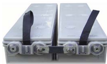
Figure 5 Battery Interconnect Bars and Hardware
