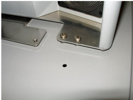
Inverter lower mounting screws installed
