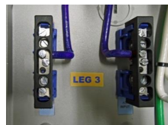
Completed. Red wires replaced with blue and "LEG 2" Sticker replaced
