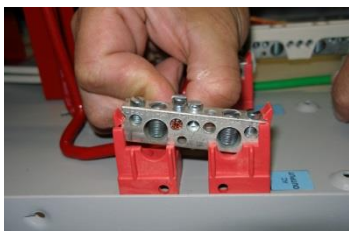
Finish removing the terminal block
