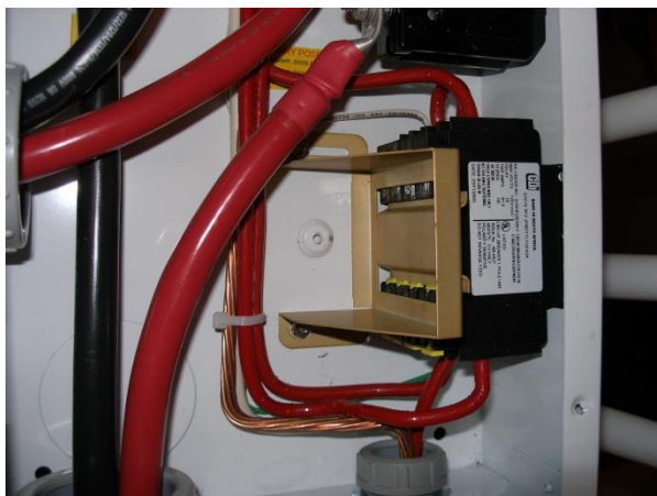
Din Rail mounted breakers
